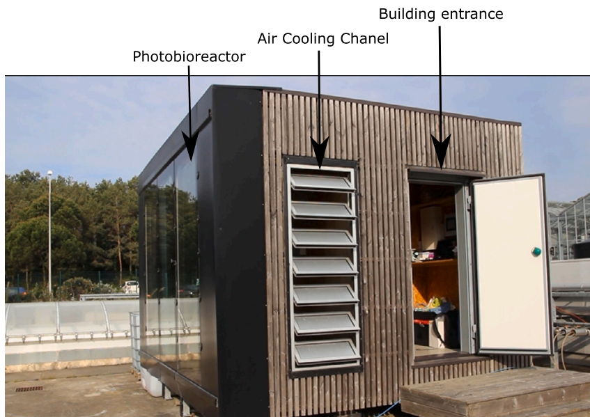
Fig. 1. Photo of the SymbioBOX pilot with location of the Air Cooling Chanel (ACC).
