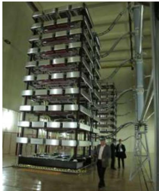
Figure I-5: Thyristor tower of the France-England connection on the french side
