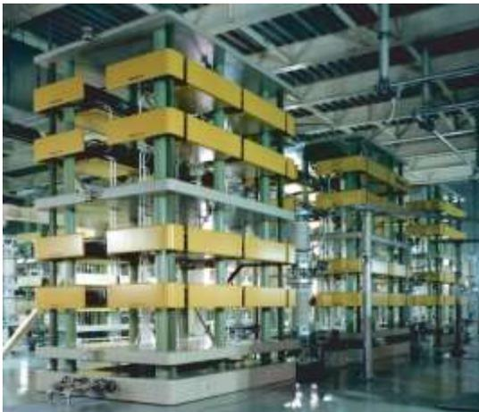
Figure I-4: thyristor tower for the frequency converter on Shin-Shinano side
