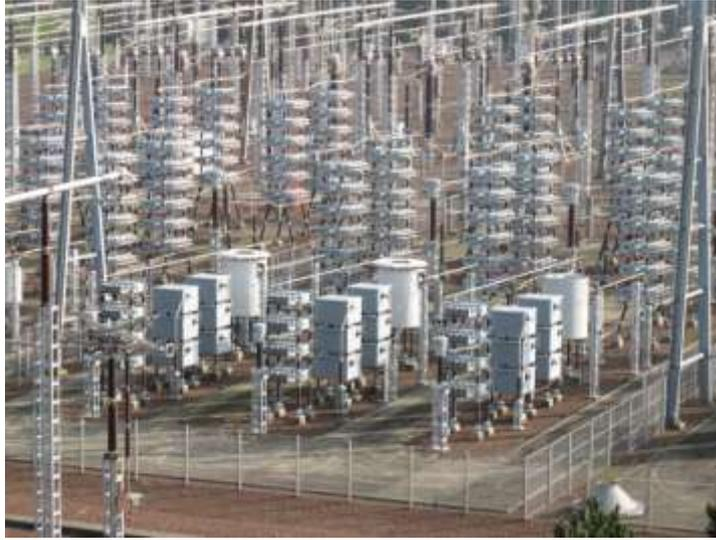
Figure I-42: LC shunt filters at « Les Madarins » converter station in France - England Interconnection
