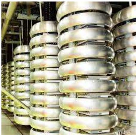
Figure I-7: Typical series valve tower of ABB
