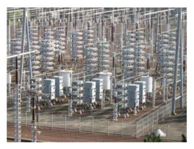
Figure I-42: LC shunt filters at « Les Madarins » converter station in France - England Interconnection
