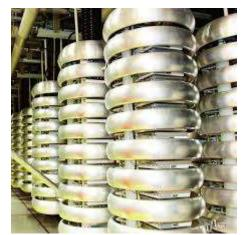
Figure I-7: Typical series valve tower of ABB
