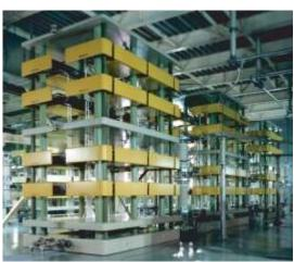
Figure I-4: thyristor tower for the frequency converter on Shin-Shinano side
