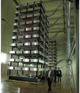
Figure I-5: Thyristor tower of the France-England connection on the french side
