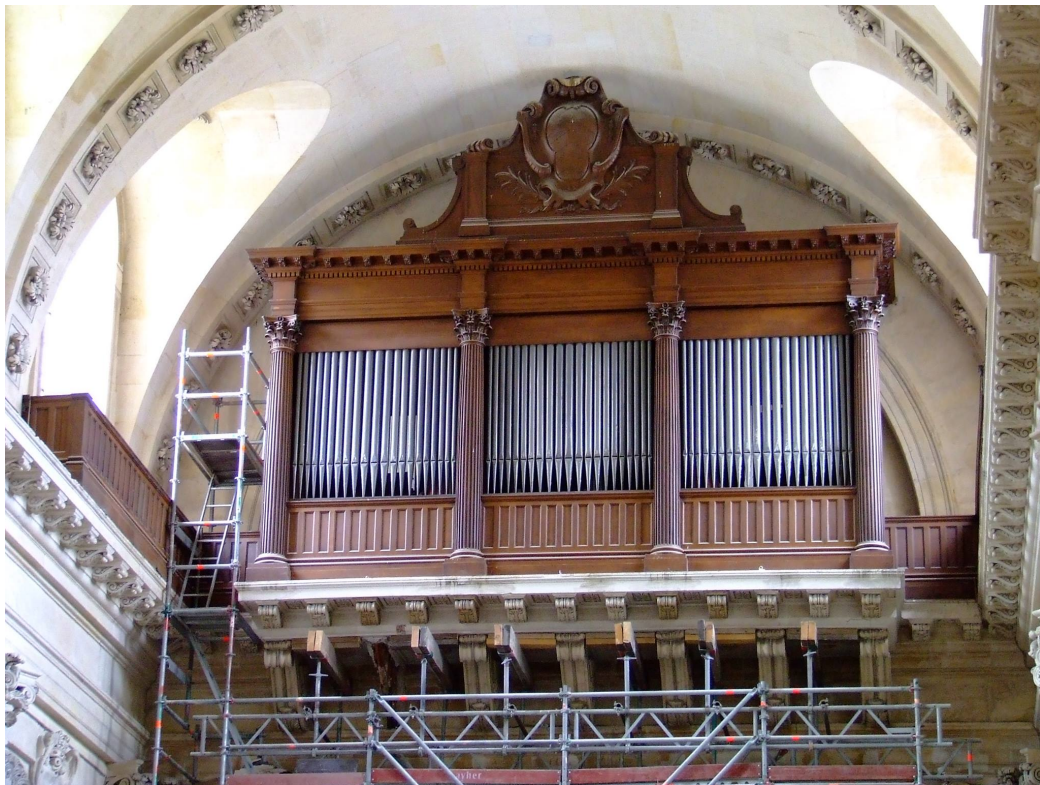
Figure 1.7: Tribune of Dallery organ in Chapelle Sorbonne supported with scaffolding. Image credit: J.-J. Soin, 2012.
