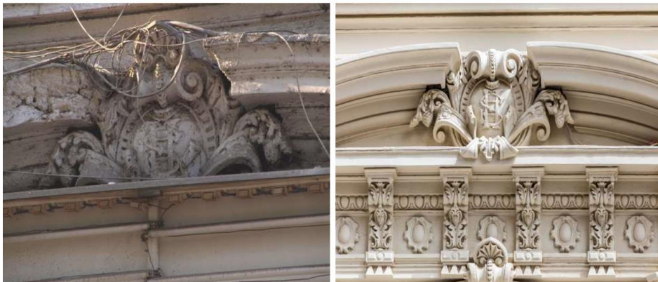
Figure 64: The state of the decorative elements before and after restoration work. Source: Al- Ismailia Company
