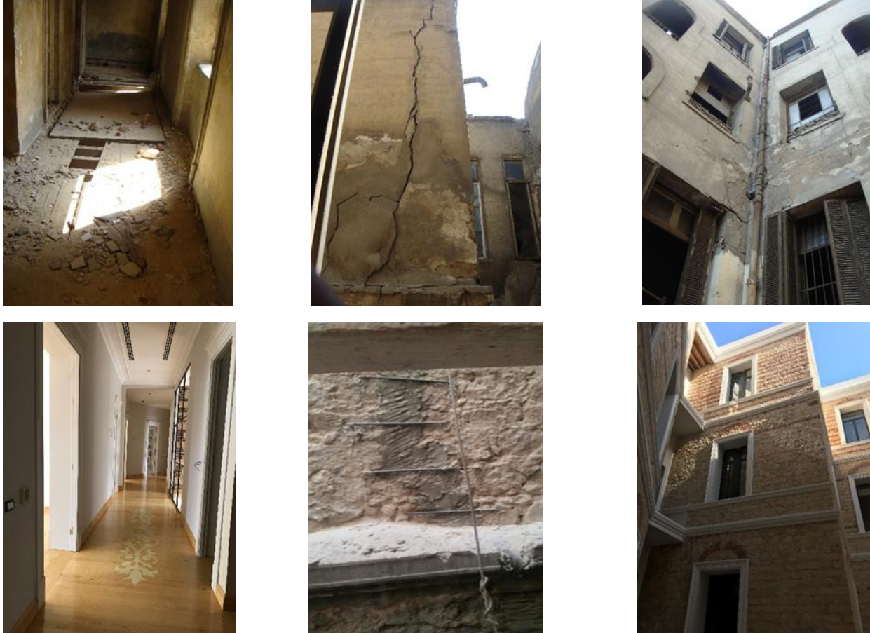
Figure 62: The exterior state of the building. Source: Al-Ismailia Company
