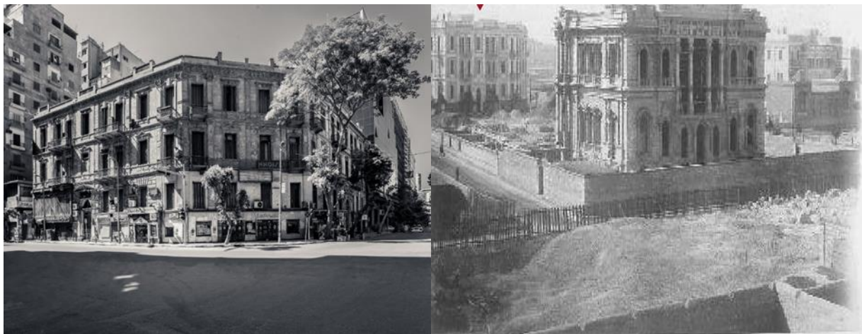
Figure 60: Old photos for La Viennoise building. Source: Al-Ismailia company for real estate investment.
