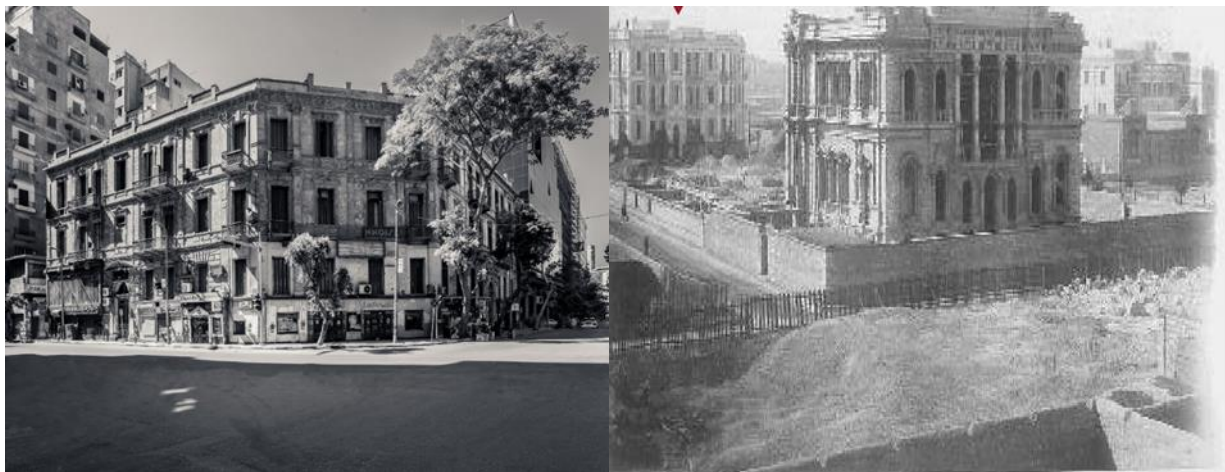
Figure 60: Old photos for La Viennoise building. Source: Al-Ismailia company for real estate investment.
