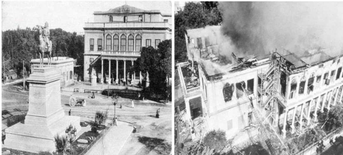
Figure 29: Opera house wooden structure turning into ashes after the devastated fire. Source: (Romany, 2019)
