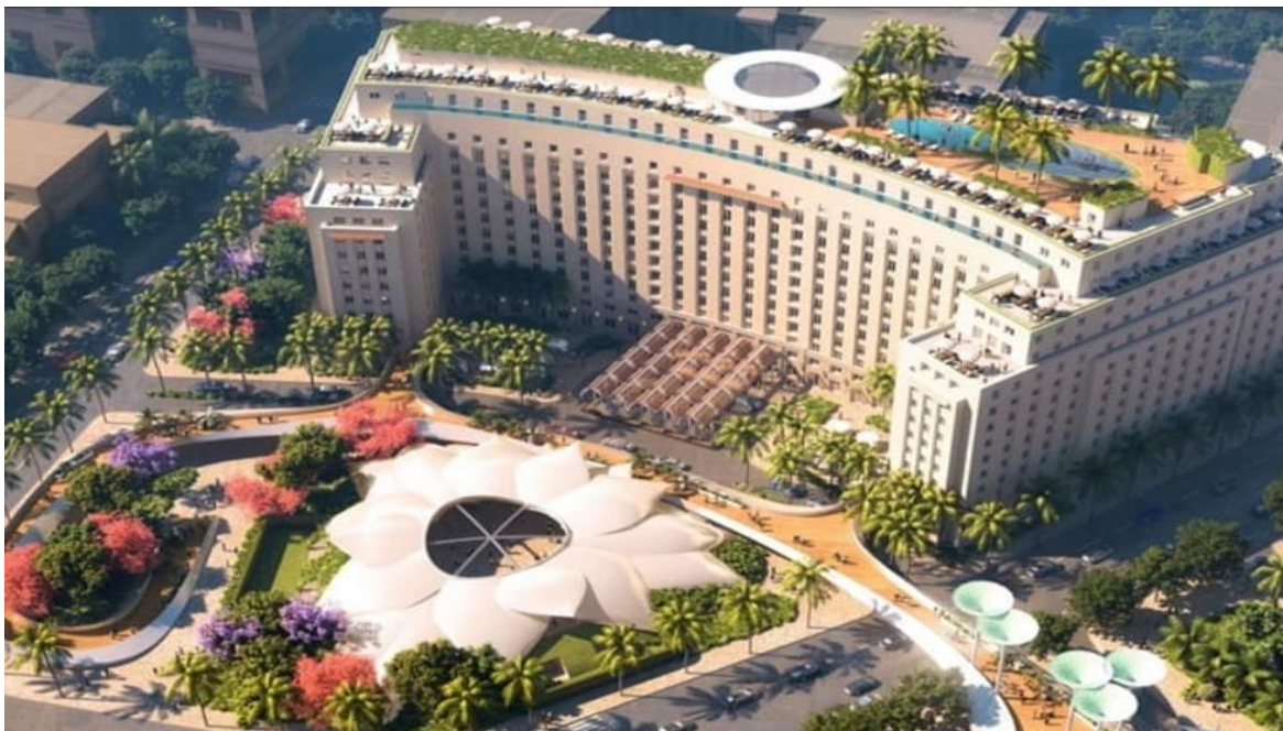
Figure 100: The suggest renovation plan for Tahrir complex. Source: (Nile FM Staff, 2021)
