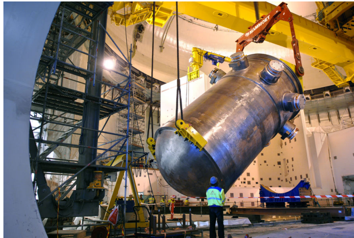
Figure 1.2: Picture of the Reactor Pressure Vessel of the Finnish European Pressurized Reactor [125], ©Areva
