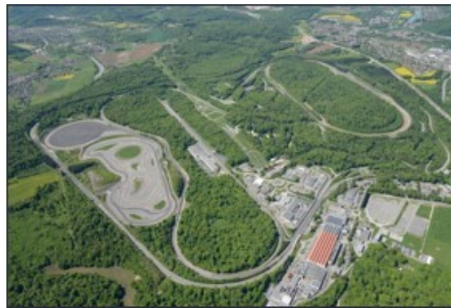
(a) PG facility
