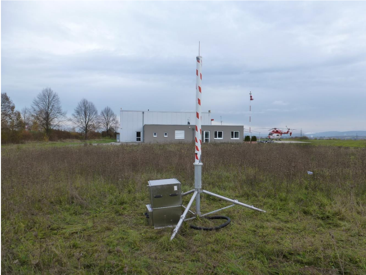
Figure 23 – MLA antenna and reflector building in Pattonville airport
