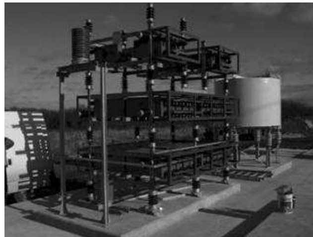
figure I.19 : Filtre shunt C_{sh} - L_{sh}
