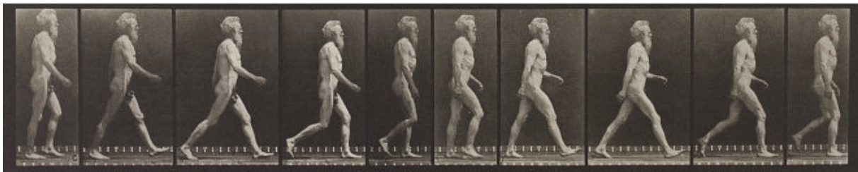
Figure 1.3: The cycle of locomotion is clearly shown in this sequence of a man walking: the single foot support stance, the double support stance and the transitions between. The coordination between arms and legs is also clearly observed. Picture from [Muybridge 1979].
