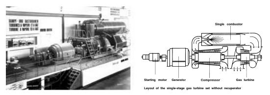
Figure 1.4: Neuchâtel first industrial gas turbine
