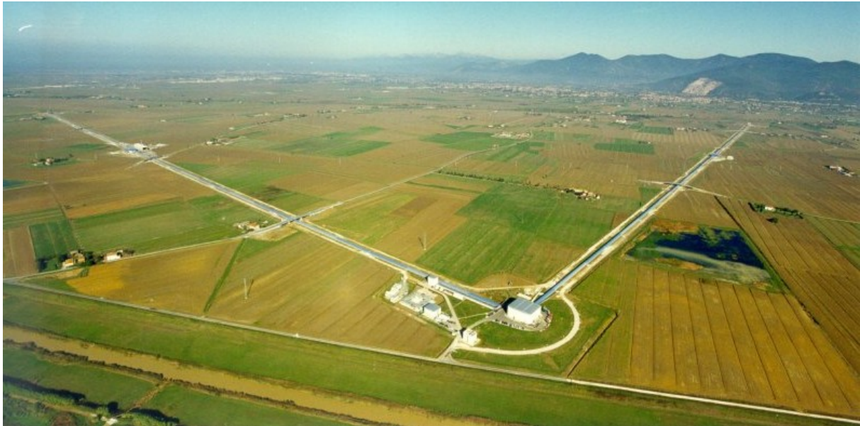
Figure 2.1: Aerial view of the Advanced Virgo+ interferometer.
