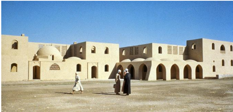
Figure 84: Village New Gourna, Hassan Fathy (1952). Source : entreprise.press/stories/2021/06/28/building-better-46142/
