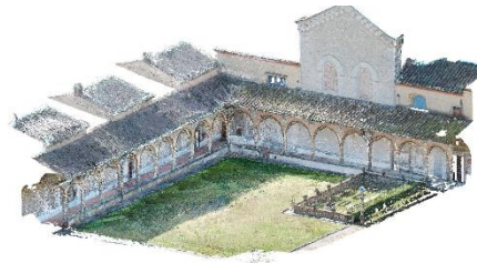
c) Photogrammetric Point Cloud
