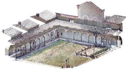
a) TLS Point Cloud
