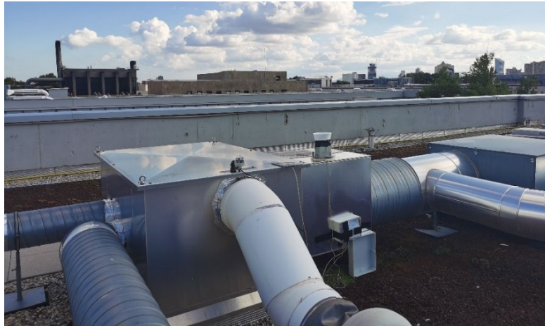
Figure 5-15. Third low-cost rainfall monitoring station trial operation location.
