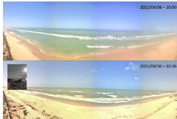
Figure 3.4: Images acquired with the camera (see Figure 2.1 for location) on the indicated time. A small picture (bottom panel, on the left) shows the ongoing construction of the riprap (from (Taveneau et al. , 2022)).
