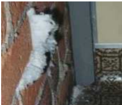
Figure 26. Images of efflorescence at the surface of a brick wall (images from google images)
