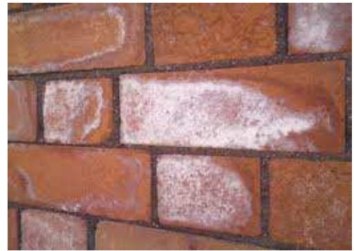
Figure 26. Images of efflorescence at the surface of a brick wall (images from google images)
