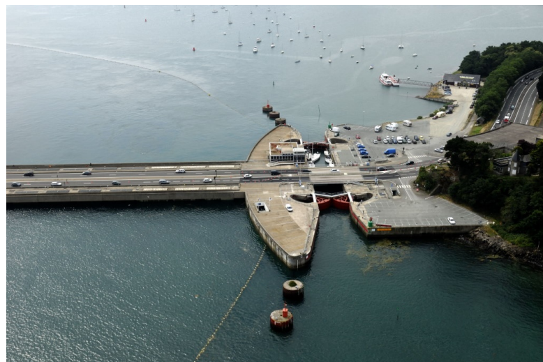
Figure 1.7 La Rance tidal power plant (Photo Credit: EDF).
