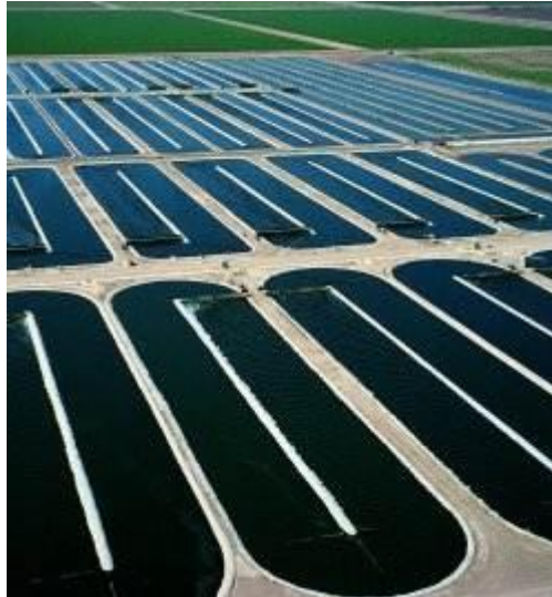
Figure 70 Raceway type culturing of micro algae for biofuel production (source: www.geni.org)
