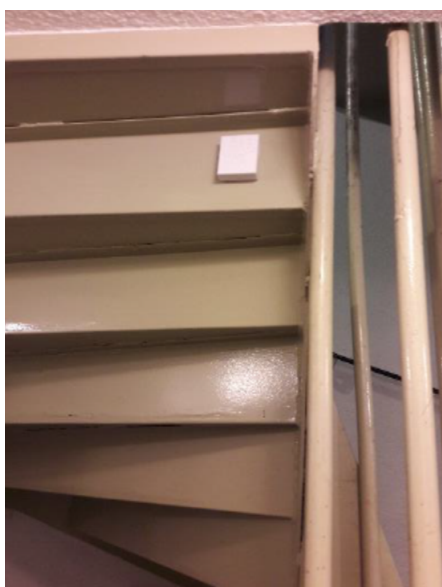
Figure 2.8: Temperature and humidity sensors installed in the buildings shared areas.
