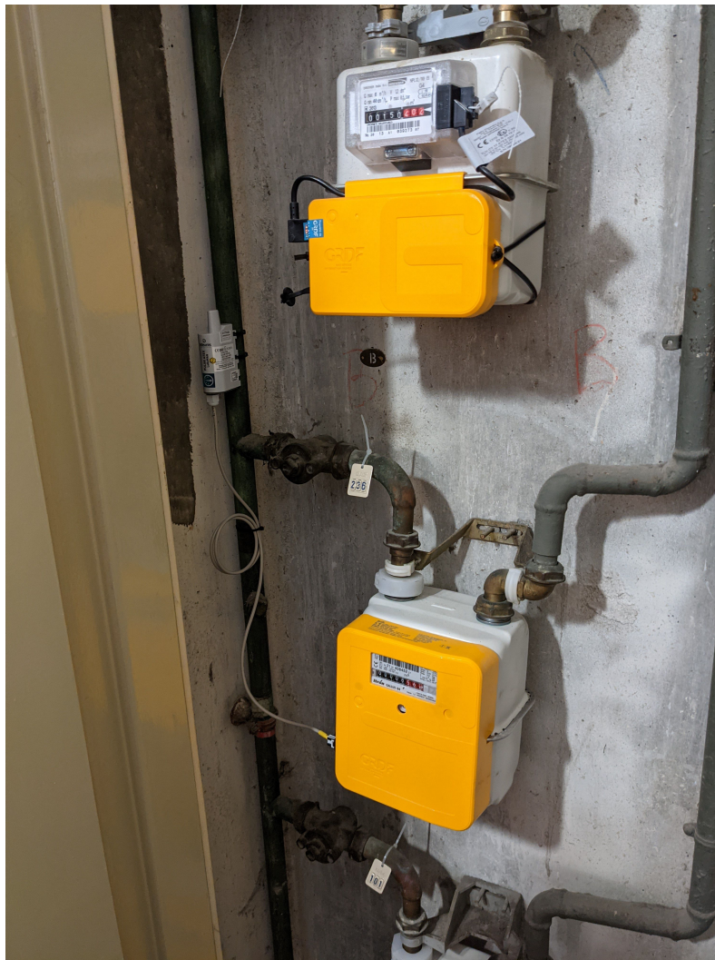
Figure 2.7: Pulse sensor for natural gas Gazpar meter.
