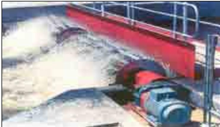
Figure (1.10): Low speed horizontal flow aerator (Twin mini rotor aeration, (Botjheng Water Ltd.).
