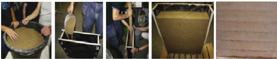
Fig. 1.1. The process of layer-by-layer RE construction [9].
