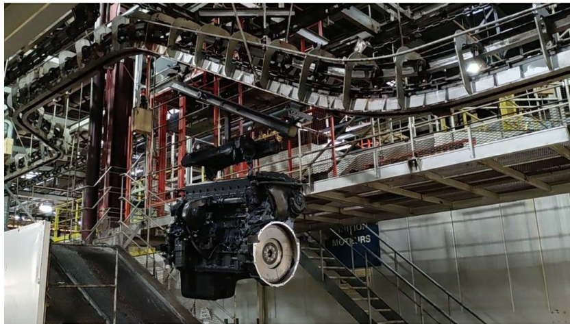
Figure 80. An engine lifted in the conveyer chain
