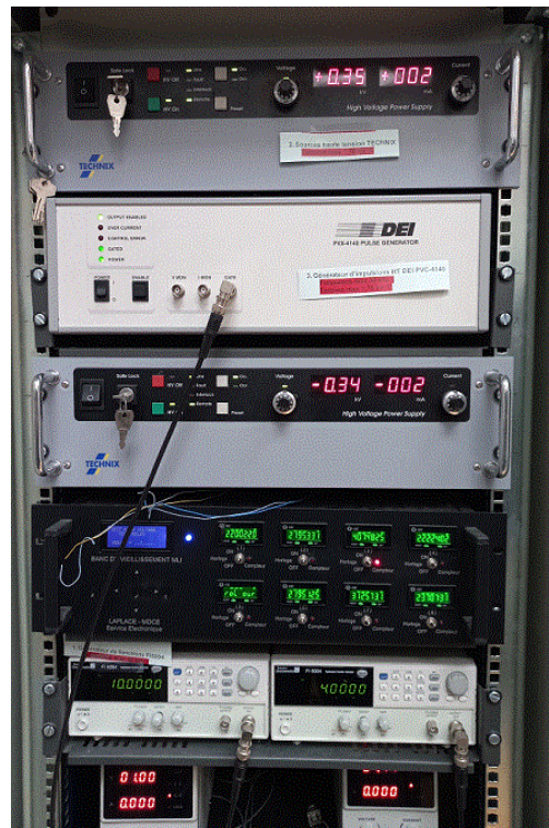
Figure 3-4 The test bench, inverter style voltage emulator [44].
