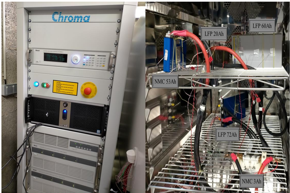
Figure IV.6 Experimental setup and tested batteries inside the climate chamber.
