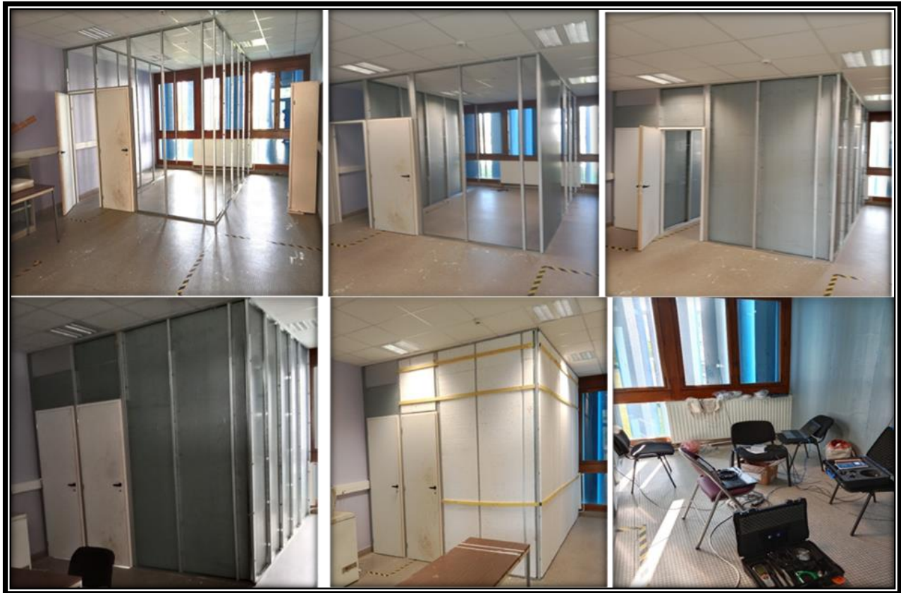
Figure 12: Pictures showing the stages of constructing the experimental-cell
