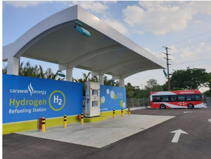
Figure 1.1: Sarawak first integrated hydrogen refueling station and hydrogen bus (Sarawak Energy, 2020)
