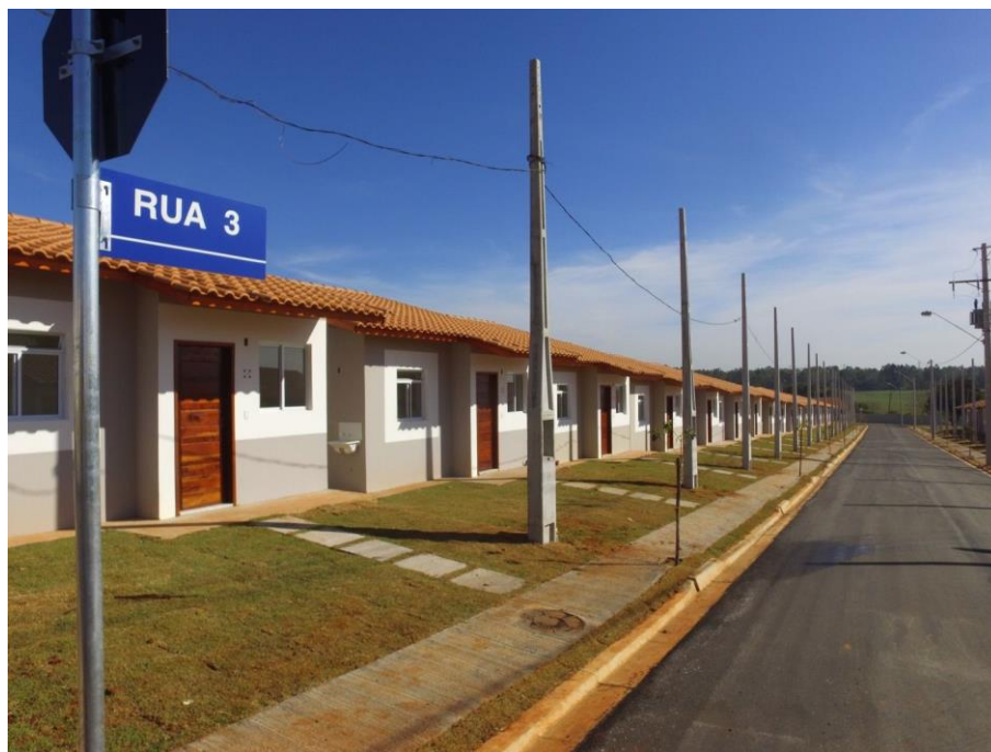
Figure C.5 – Residencial Estoril, 360 maisons (124-200m 2 ), Sorocaba – SP (Magnum 2020)
