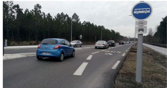
An example of reserved lane to carpools and buses
