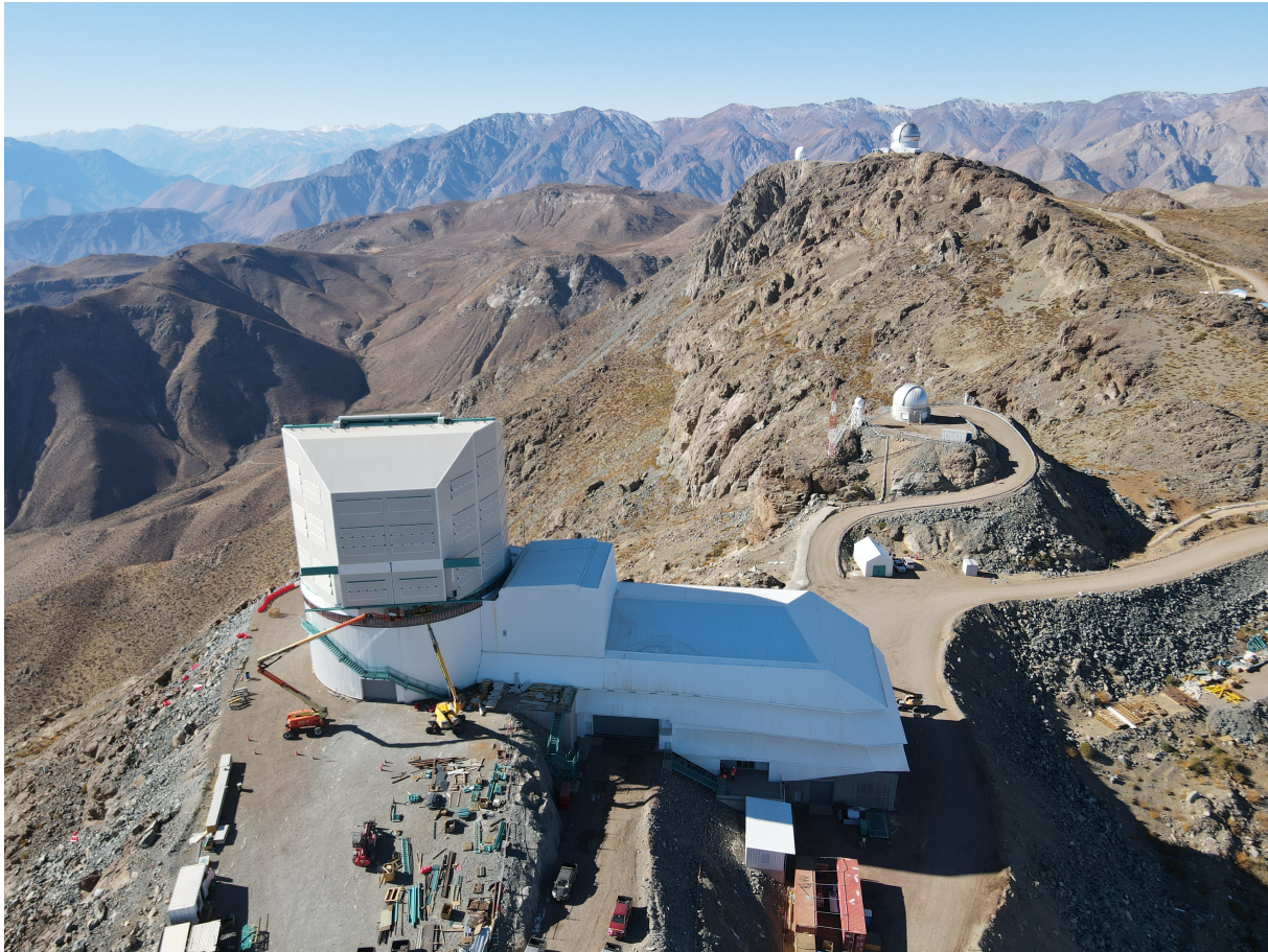
Figure 3.1: The Vera Rubin observatory under construction. Credits https://www.lsst.org/ .
