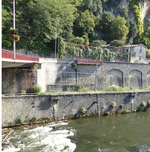
Figure 3.2: Example of a retaining wall.
