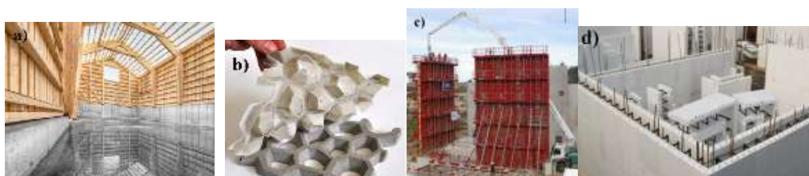
Figure 2; a) Wooden formwork ©123rf.com, b) 3D printed Flexible Formwork ©Brian Peters, ACADIA 2014, c) metal formwork © Hussor.com, d) insulating concrete formwork © theconstructor.org
