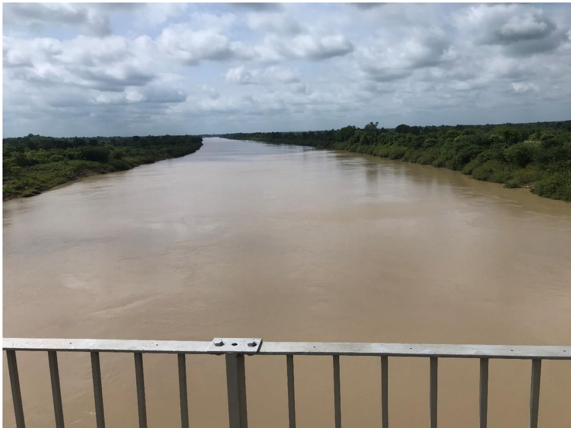
Figure 4. 11: A section of the White Volta from the Ntereso- Yapei bridge.
