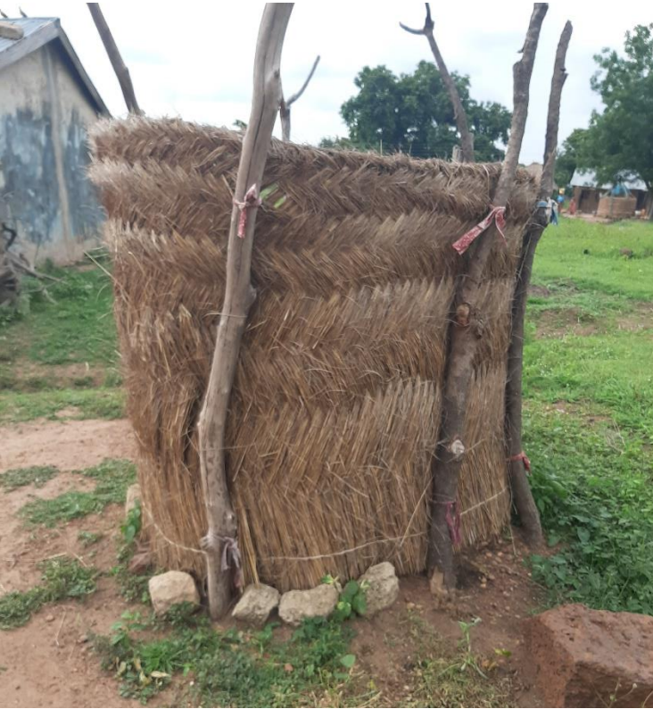
Figure 4. 25: Woven straw mat at Ntereso used as a covering to a urinal (may double as a bathhouse)
