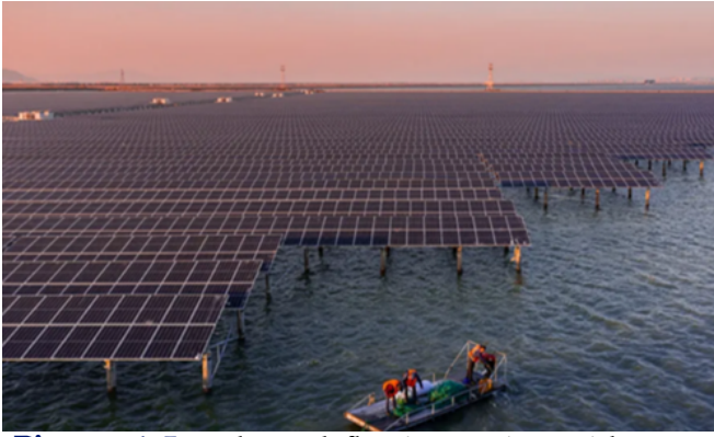
Figure 1.5 —Colocated floating project with aquaculture assets, developed by Chint Group© in China's Zhejiang province, the installed capacity reaches 550 MWp.
