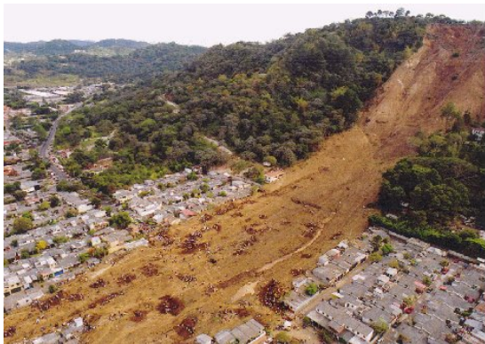
(c) Landslide following an earthquake (Las Colinas, Santa Tecla, El Salvador)
