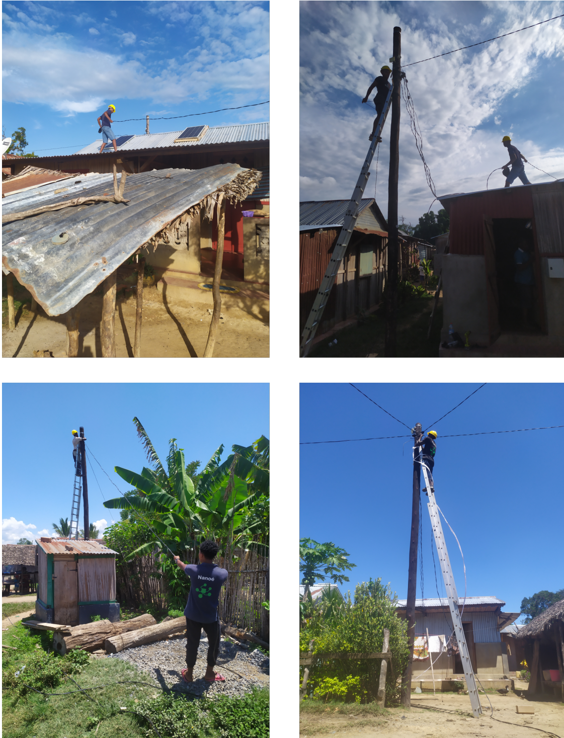
Figure IV.6: Construction work in Ambohimena.
