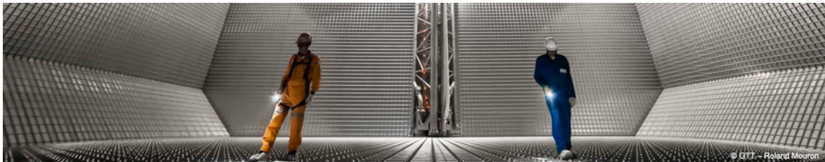
Figure 1.3: Two people working in an empty tank ship designed by GTT. This ship carries liquefied natural gas. The control network is visible on the walls of the tank.
