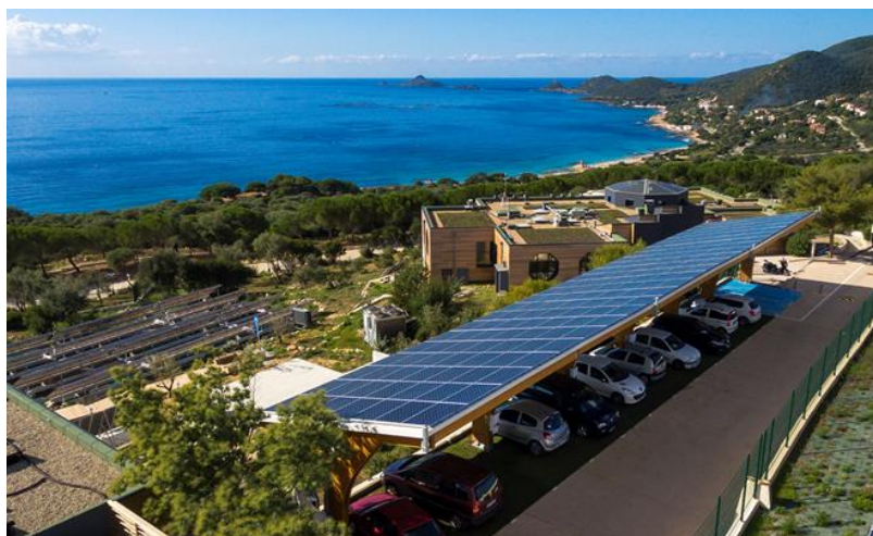
Figure 2-6 : Ombrière photovoltaïque
