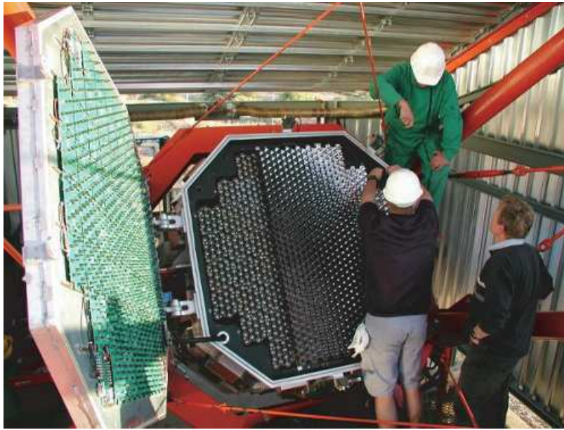
Figure 6.3: Photograph of one of the cameras of CT 1-4 during the installation of Winston cones
