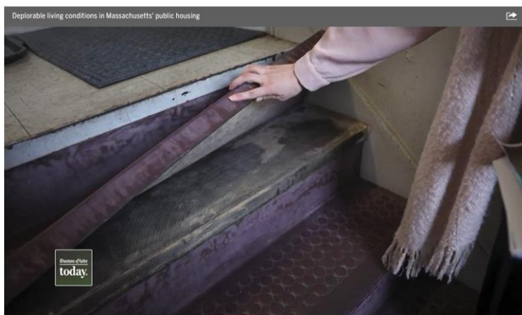
Housing reporter Andrew Brinker sheds light on the lack of funding for Massachusetts' public housing.
