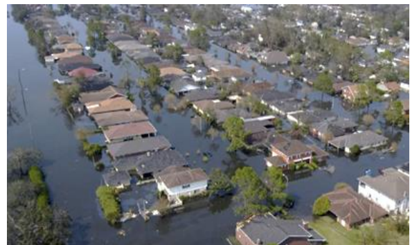
Figure 2-1 Aerial view of damage, Courtesy of Wikimedia Commons
