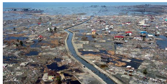
Figure 2-20 A coastal view in Banda Aceh after two weeks from the tsunami, (Prasad, 2019)
