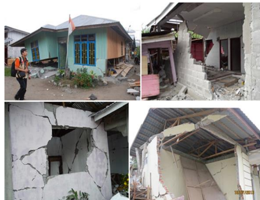
Figure 2-29 pictures of damaged houses after the 2013 earthquake, (Okazaki,2014)
