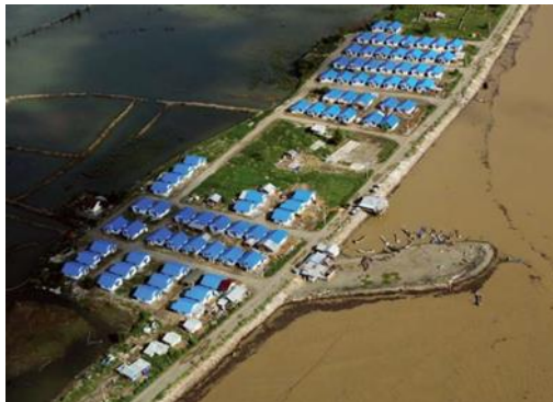
Figure 2-31 houses built in proximity to the riverside in Alue Naga, (NAD-Nias,2009).
