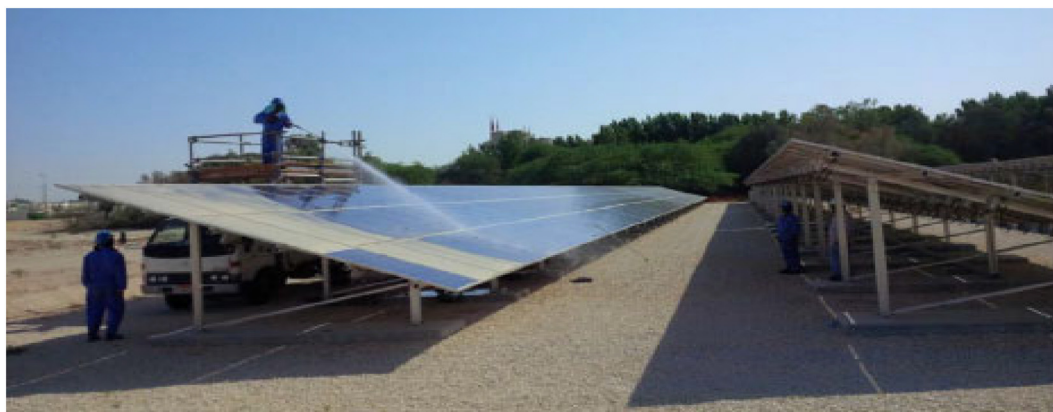
Fig. 8. Cleaning process for PV panels (Alnaser et al., 2018).
