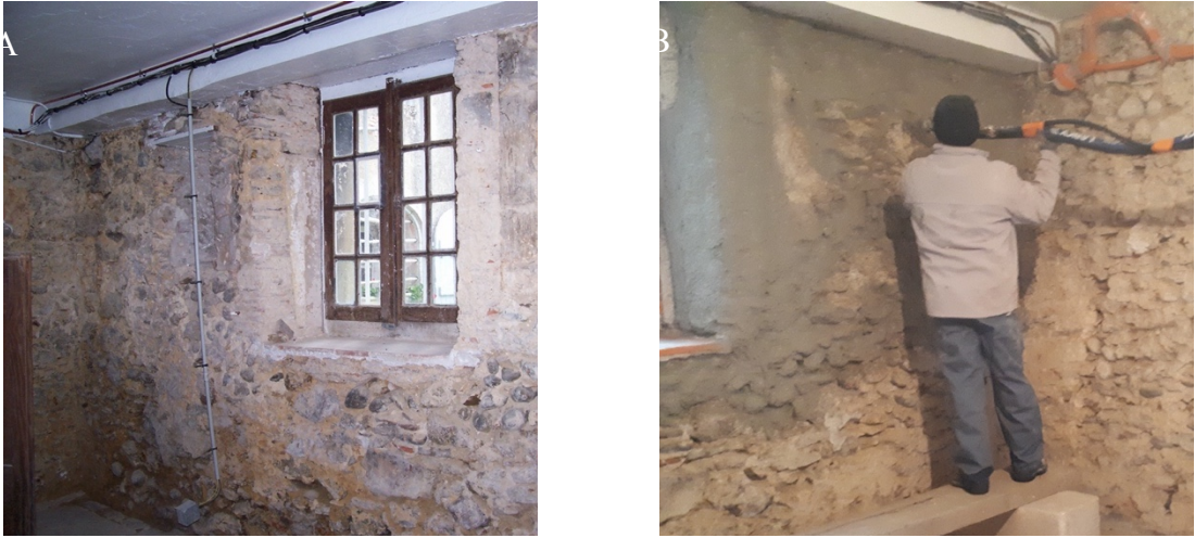
Figure 104. Image of the wall before the hemp mortar insulation (a) and the application process (b)
