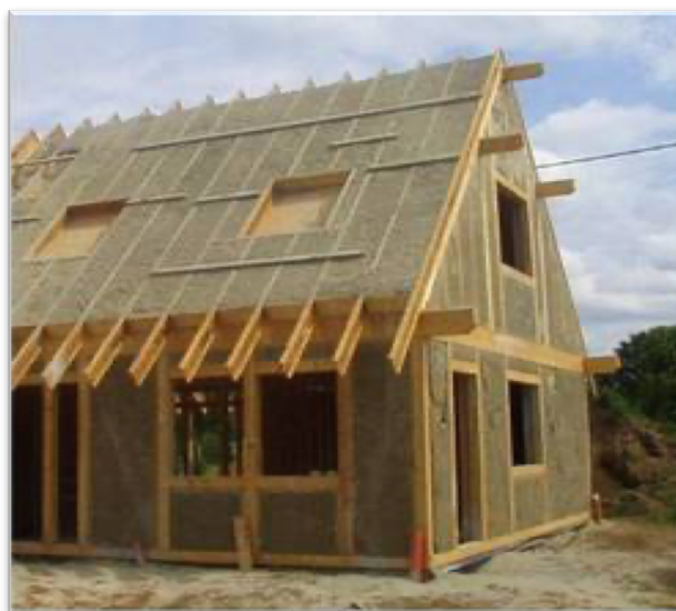
Figure 10. Different application of hemp mortars in construction (roof and wall insulation) (Chabannes et al., 2018)
