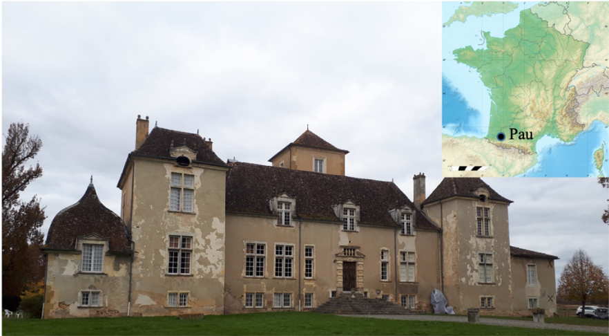
Figure 103. Study case: stone masonry castle in the region of Pau (France)
