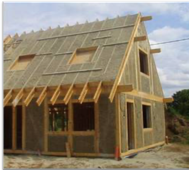
Figure 10. Different application of hemp mortars in construction (roof and wall insulation) (Chabannes et al., 2018)
