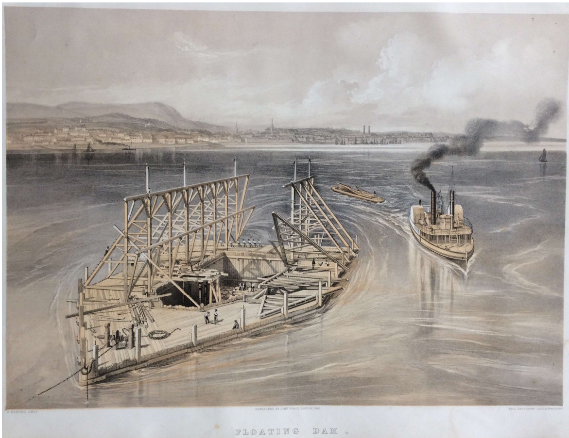
Fig. 14 Floating Dam , from Hodges, Construction of the Great Victoria Bridge , LAC, Winkworth Collection, R9266 Vol. 4107
