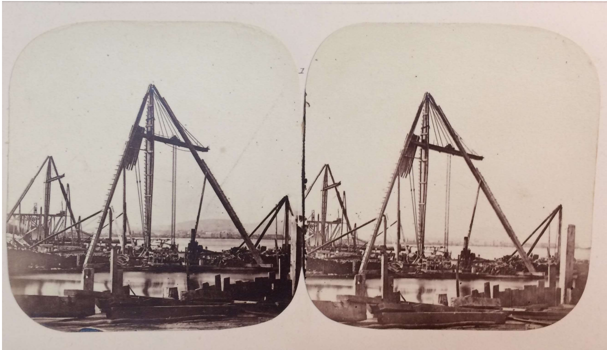
Fig. 17 Coffer Dam previous to Pumping , Notman, n.d, Photograph, McCord Museum, N-0000.193.147.155
