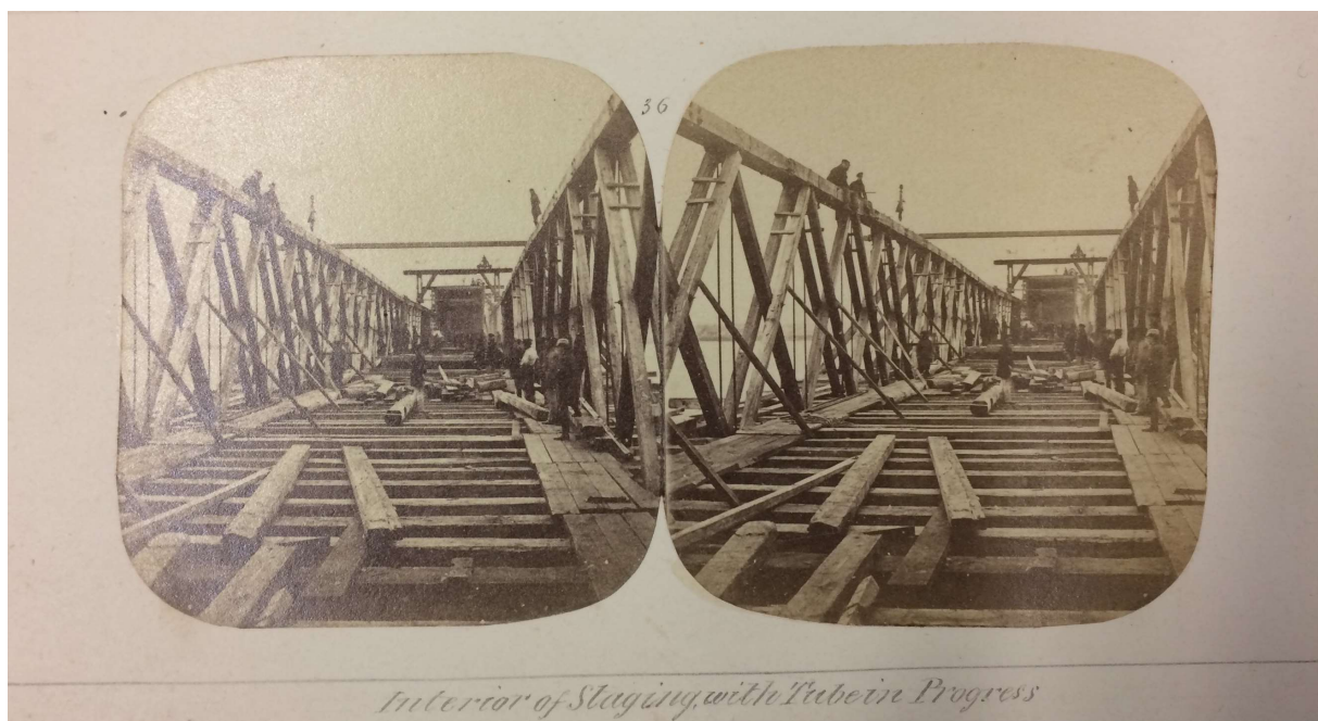
Fig. 42 Interior of Staging with Tube in Progress , William Notman, LAC, Joseph Patrick Books collection, PA-187238, ca. 1859.
