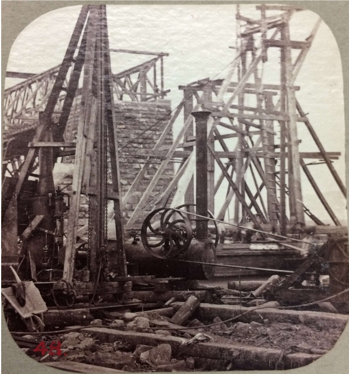
Fig. 34 Floating Derrick and Pile Driver , Notman, n.d., LAC, Merrilees, 1980-149_55073.1, 2000805 724, No. 1 p.16
