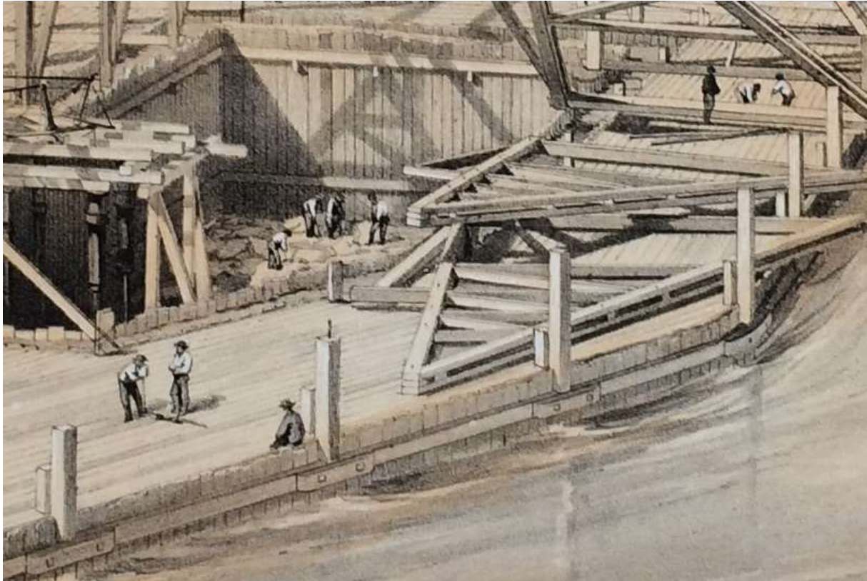
Fig. 15 Enlargement Floating Dam , from Hodges, Construction of the Great Victoria Bridge from LAC, Winkworth Collection, R9266 Vol. 4107
