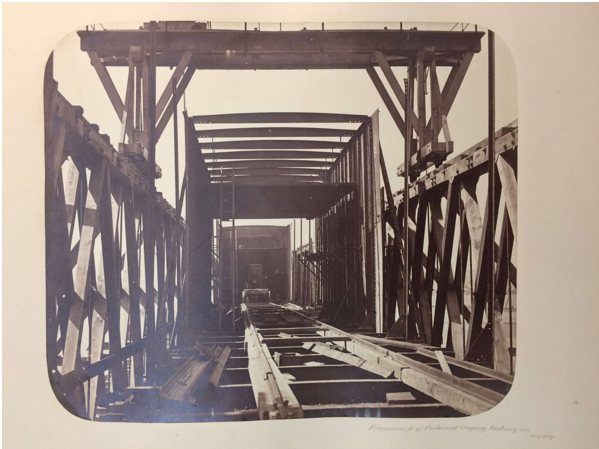
Fig. 28 Framework of Tube and Staging Looking In , Notman, May 1859, McCord Museum, N-0000.193.132-133
