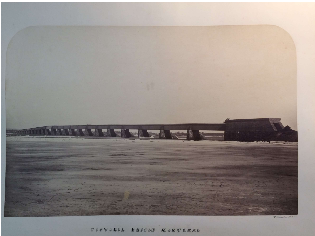
Fig. 1 Victoria Bridge Montreal , William Notman, McCord Museum (Montreal), N-0000.193.183, 1859-1860
