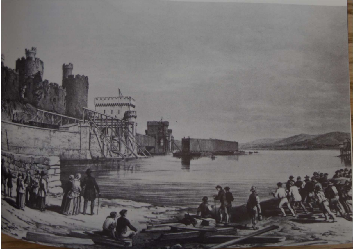
Fig. 25 Conway . Floating the second tube into position, 12 th October 1848, unknown artist, from Millar, William Heap and his Company, 29
