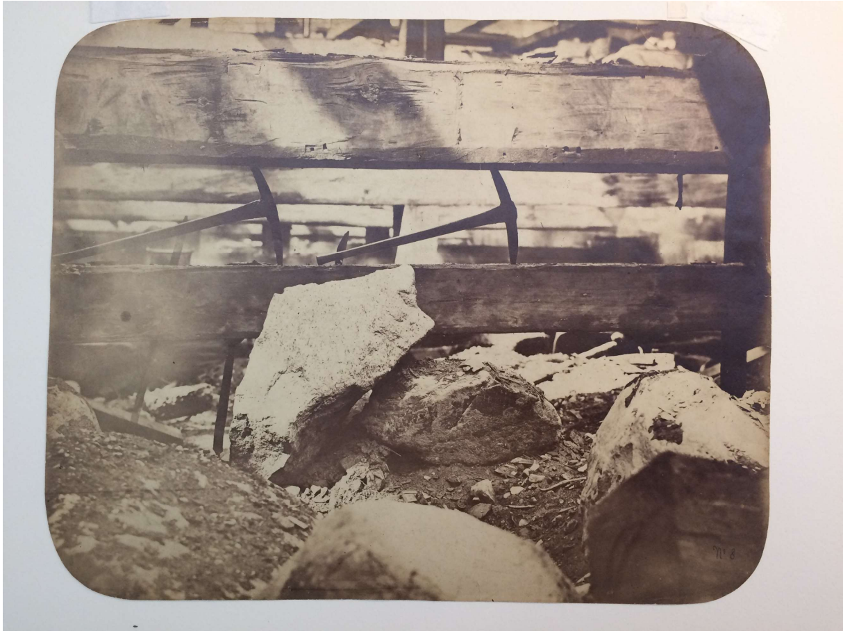
Fig. 9 Untitled , Notman, n.d., McCord Museum, Box 'William Notman the founder', N-0000.392.2.28 Pickaxes left in a wooden structure, maybe a dam, with boulders that might need to be removed.
