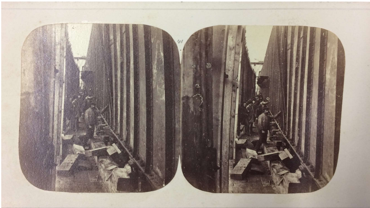
Fig. 11 View of down stream side of No. 12 Tube from No. 11 Pier, showing displacement of Longitudinal and Packing, November 9 th , 1859, 9 Nov. 1859, Notman, LAC, PA187234
