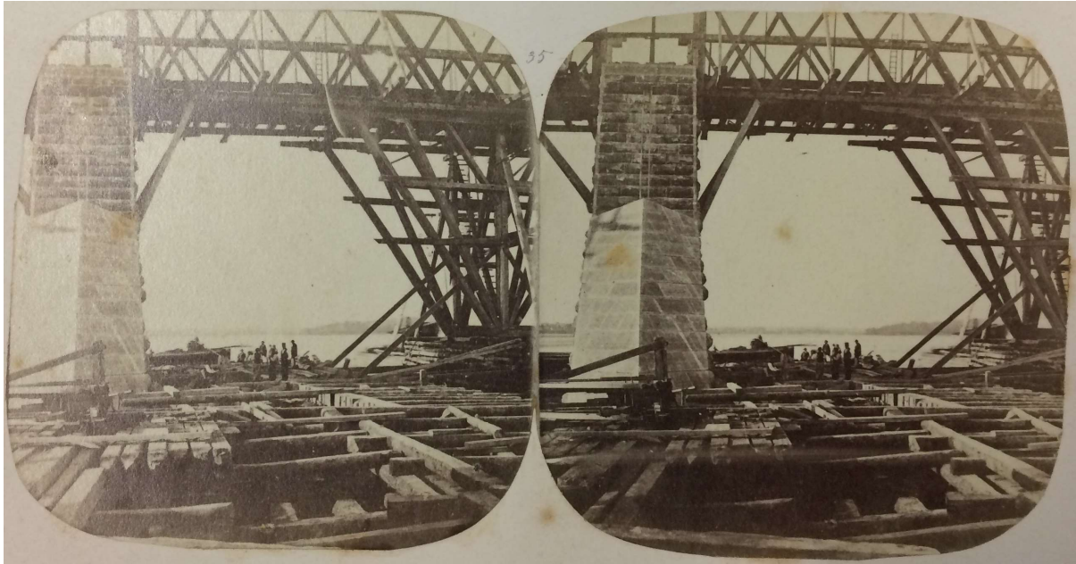
Fig. 27 No. 11 Pier Showing Cutwater , Notman, n.d., LAC, Books, Joseph Patrick, 1983-600006, 20000629894, 1858-1860, no PA number
