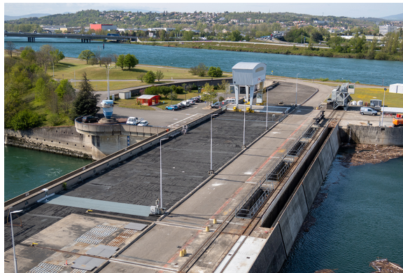
Figure 1.1 – Example of a CNR run-of-the-river hydroelectric power plant (location: Pierre-Bénite, France).
